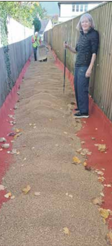
Dumping and spreading gravel over the newly-laid tennis carpet. Photo: Bob Merry
