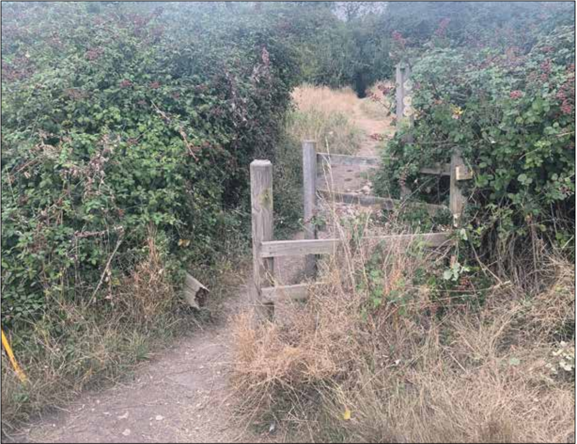
A dilapidated timber kissing gate prior to removal and replacement with a steel pedestrian gate.
