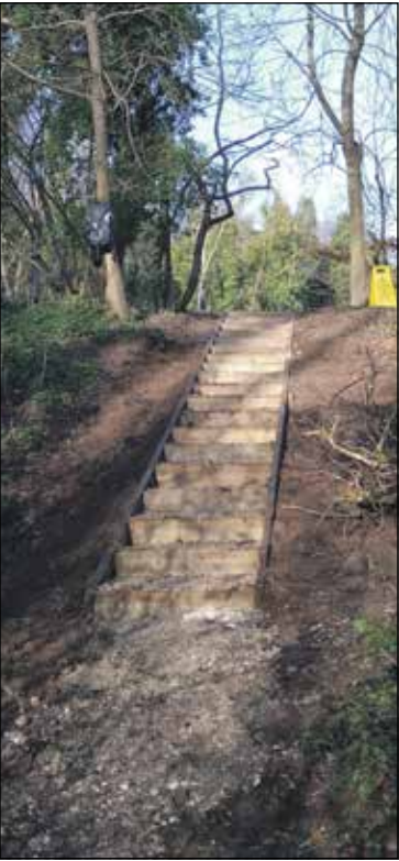
The finished flight of steps. Photo:Wim Klaucke
